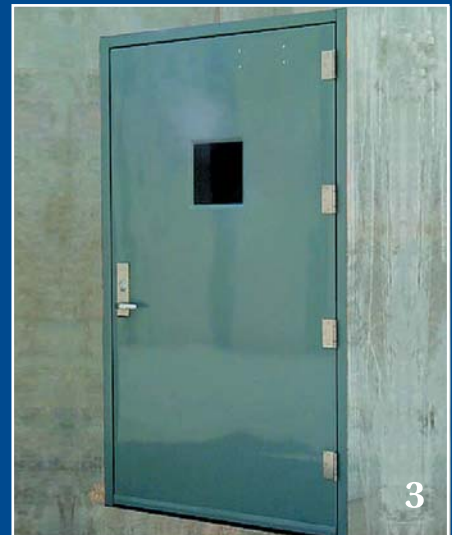
(3) Remove Straps – install anchors
